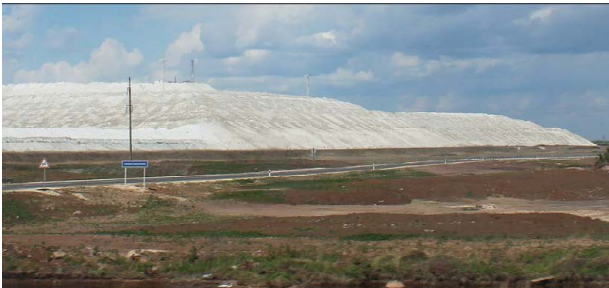
Figure 9. Large Phosphogypsum Storage Site in Florida (source: IPNI-2019)
